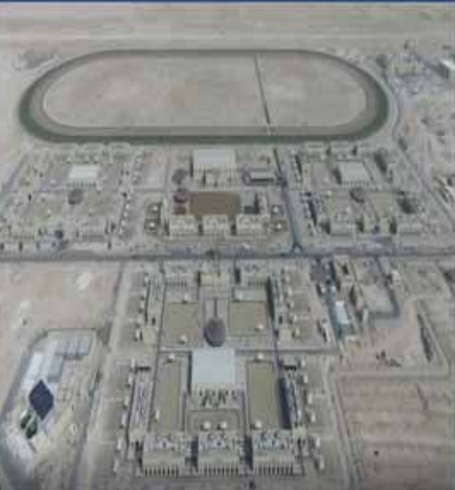
CONSTRUCTION OF HORSE OWNER'S COMPLEX AT AL KHOR-PHASE II
