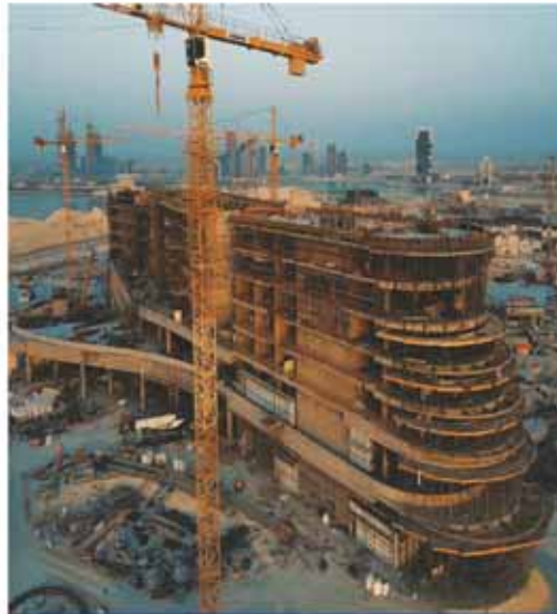
QETAIFAN ISLAND NORTH PROJECT PHASE 1- PACKAGE 5 HOTEL
